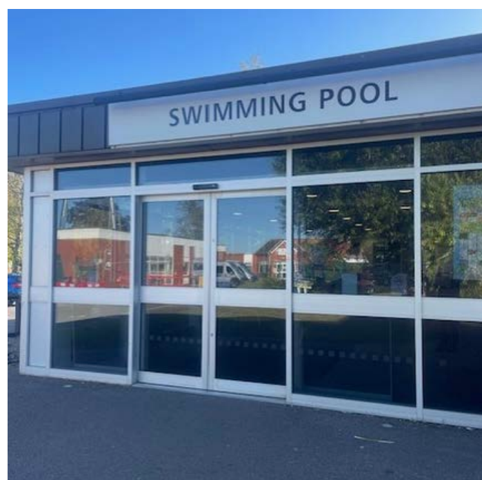
Automatic Entrance doors
