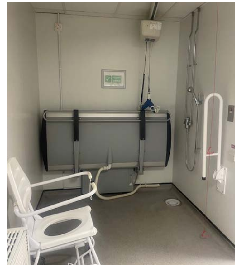
Accessible Changing room with hoist
