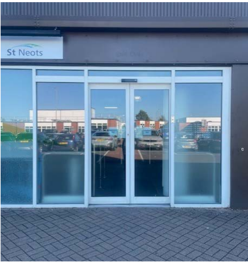
Automatic entrance doors
