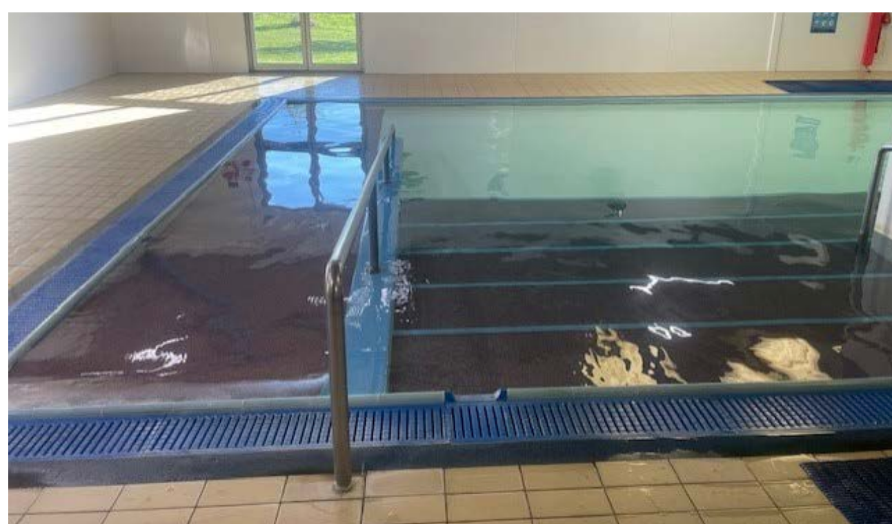
Pool Ramp and walk in stairs
